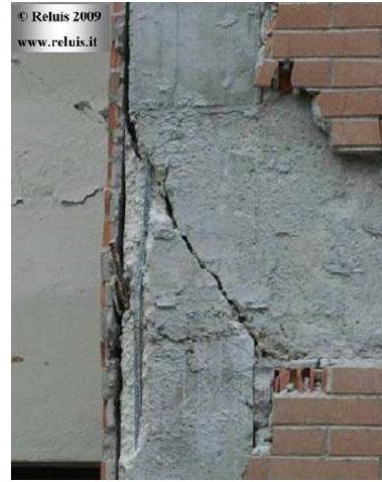
Diagonal cracking
